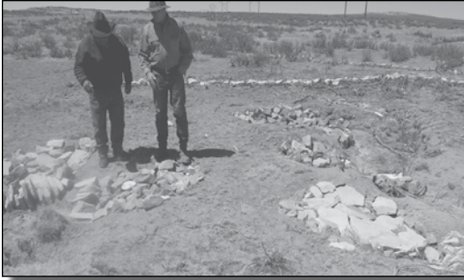
Ted Mace and Kirk Gadzia inspecting erosion control structures on Ted's allotment.
