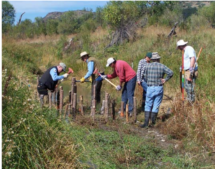
Volunteers install a picket baffle during a workshop on the Dry Cimarron, Folsom, NM, October 2005.
